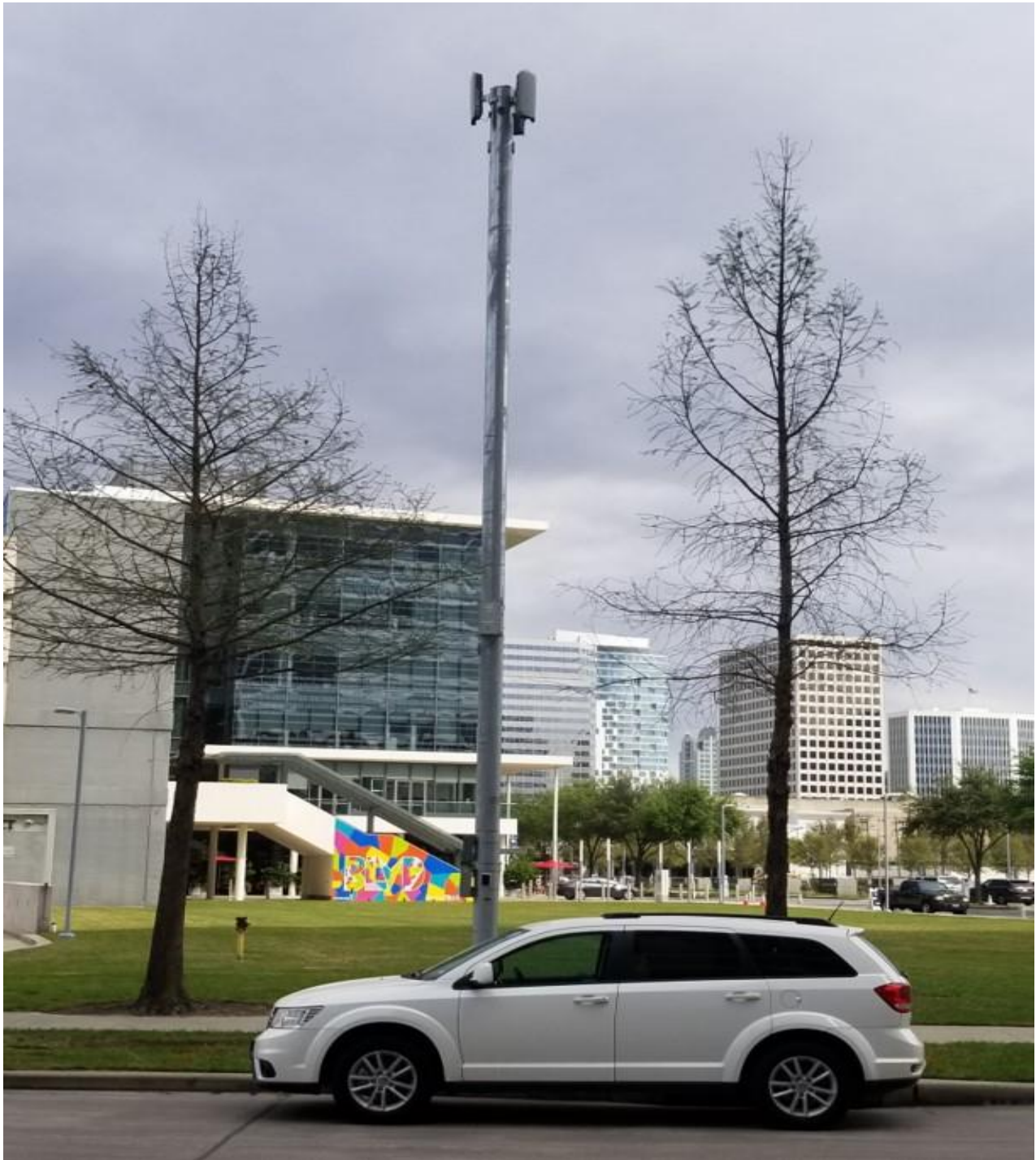
Example Small Cell Pole for Site Location Name: Katy_119.
